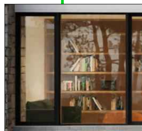
◇ Wood Windows & Sliding Doors w/ Dark Aluminum Exterior Cladding
